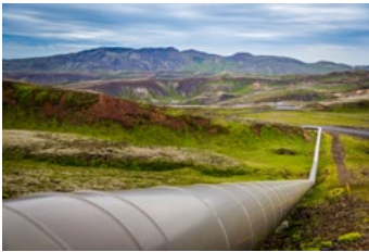
In the pipeline
